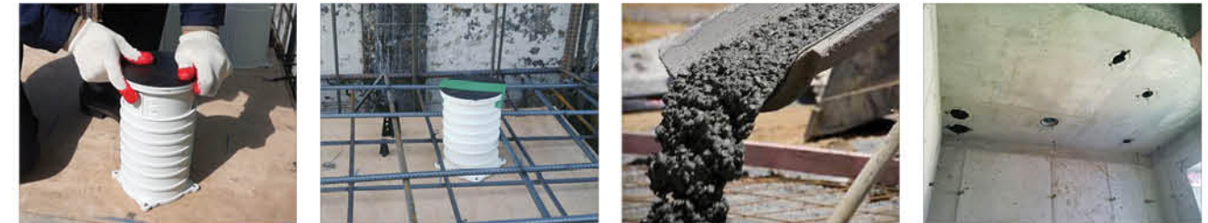
Place, Fix, Control Height
